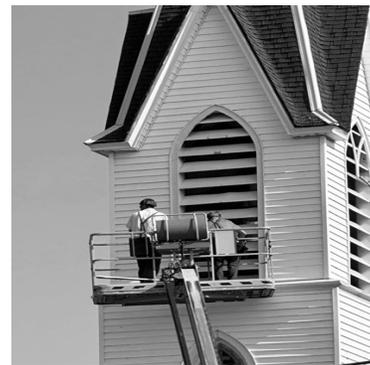
Work was completed on the outside of the bell tower by Turkey River Construction, Elgin, IA; the decorative arches were replaced, loose slats were repaired and reattached.
